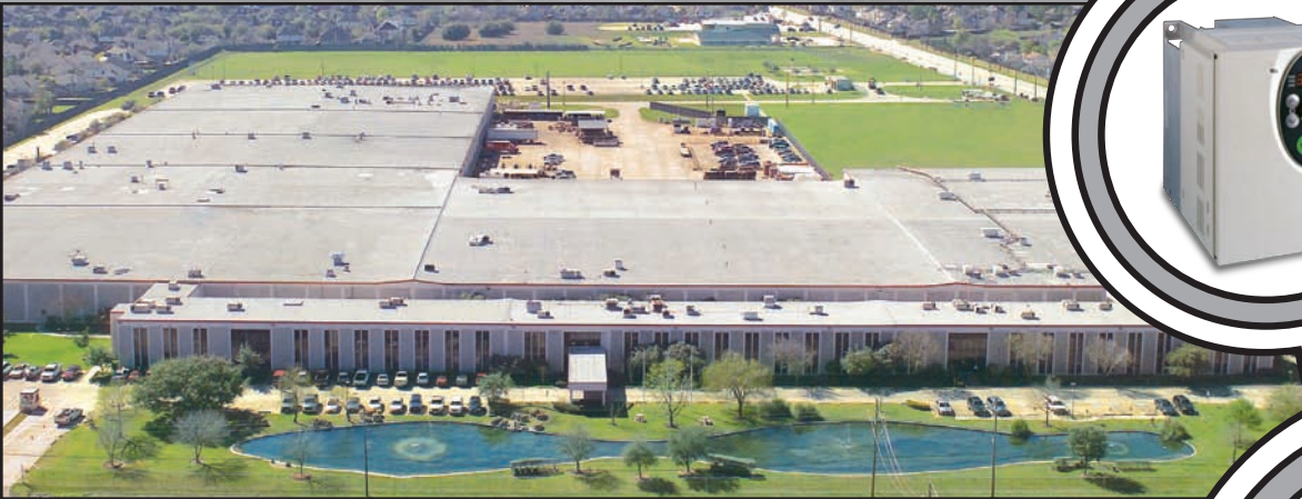
North American Headquarters & Manufacturing Facility (Houston, TX)
